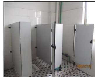
Photo of the sanitary facilities Toilet.JPG
